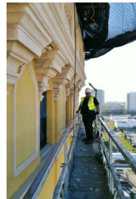
*Freedom Tower access was provided by Kaufman Lynn using fixed scaffold at top and bottom and swing stage for the tower shaft (bottom areas were accessed by self-propelled high reach). Conditions were noted using hand-held ruggedized tablets directly on CAD drawings or overlaid on original drawing scans, as required.*
