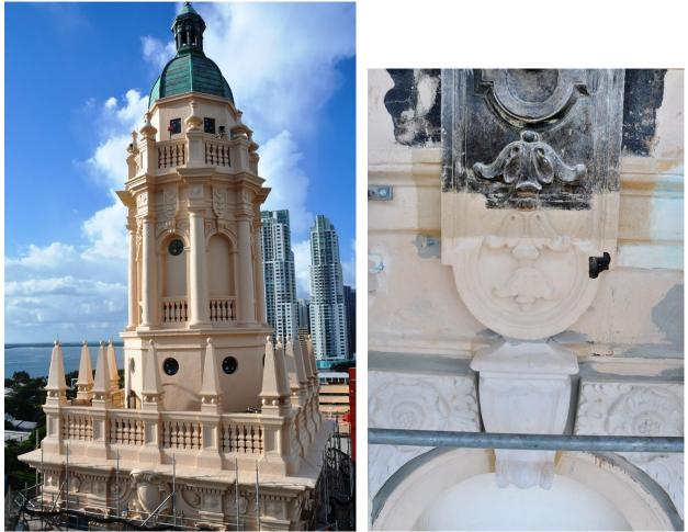
Upper tower repairs included a combination of in-kind replacement, Jahn patching, and conservation treatment.
