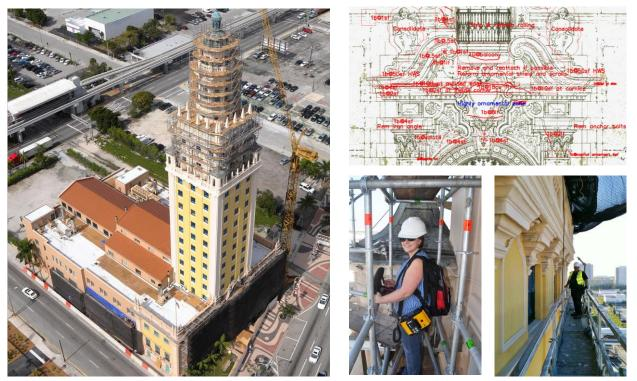
Freedom Tower access was provided by Kaufman Lynn using fixed scaffold at top and bottom and swing stage for the tower shaft (bottom areas were accessed by self-propelled high reach). Conditions were noted using hand-held ruggedized tablets directly on CAD drawings or overlayed on original drawing scans, as required.
