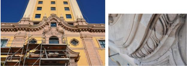
Lower level concrete was uncoated and repairs included careful cleaning and removal of biological staining, Jahn mortar patching, and selective in-kind replacement.
