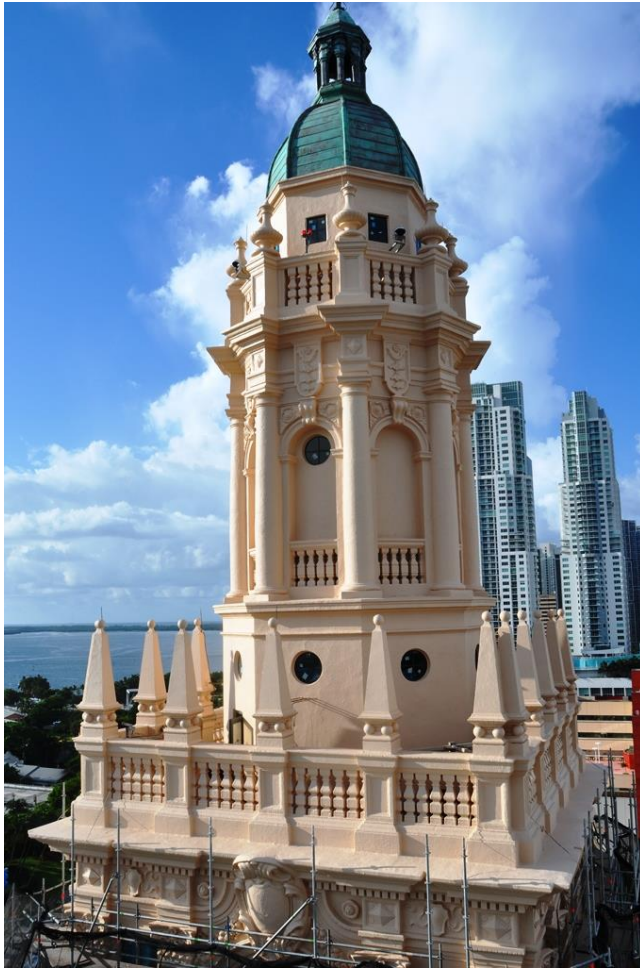
Upper tower repairs included a combination of in-kind replacement, Jahn patching, and conservation treatment.
