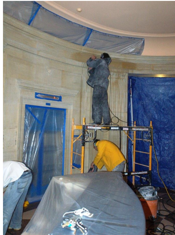
(Image Above) Extensive protection of adjacent wall surfaces was required to minimize any impact from overspray. (Below) Worker honing the wall surface with a hand-held polisher.
