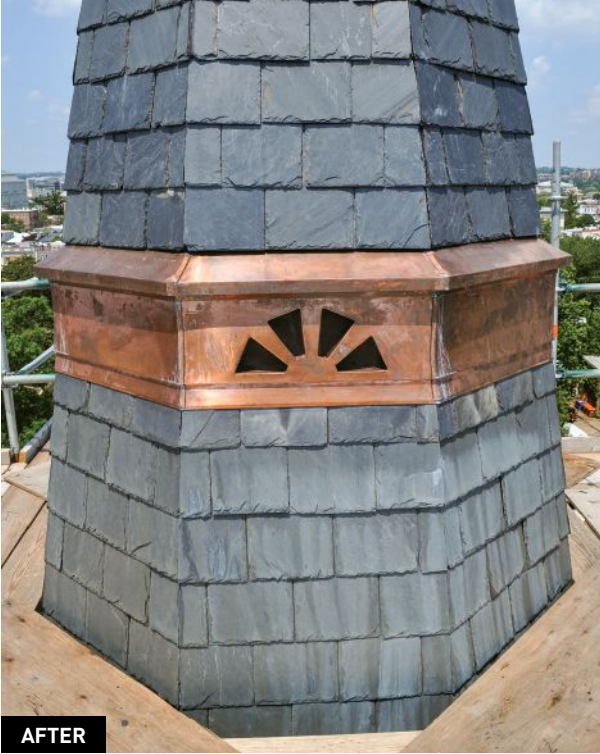
ABOVE The main tower of Mark’s Episcopal Church in Washington, D.C., had four turrets that were extensively repaired and restored by the Aeon Preservation team. This entailed rebuilding wooden framing, new copper roofing and cladding, fabrication of new decorative stones, and rebuilding large sections of masonry.
