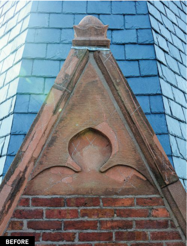
ABOVE One of the more challenging aspects of this project was trying to recreate the heavily damaged finials on the main tower. They had been patched and re-carved so many times that they no longer resembled anything like the original highly ornamental finials. The restoration team only had one historic low-resolution image to help guide the replacement.
