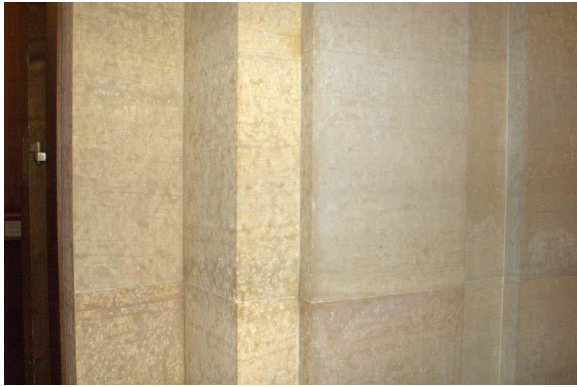
(Image Above) Left side shows honed finish, right side shows the surface prior to treatment.
