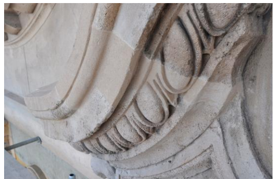
Lower level concrete was uncoated and repairs included careful cleaning and removal of biological staining, Jahn mortar patching, and selective in-kind replacement.
