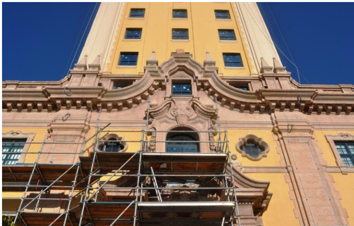
Lower level concrete was uncoated and repairs included careful cleaning and removal of biological staining, Jahn mortar patching, and selective in-kind replacement.
