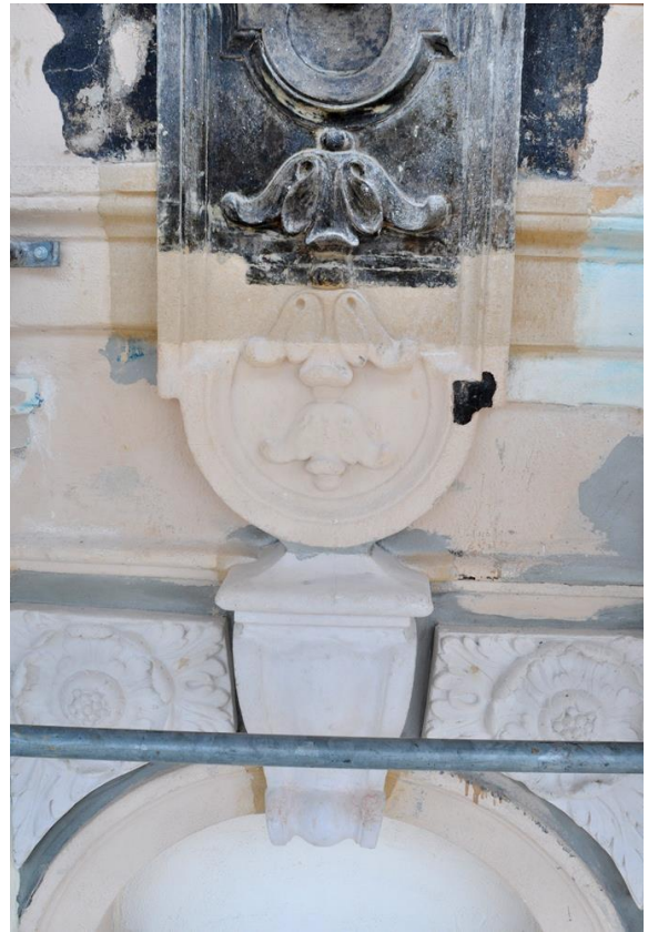
Upper tower repairs included a combination of in-kind replacement, Jahn patching, and conservation treatment.
